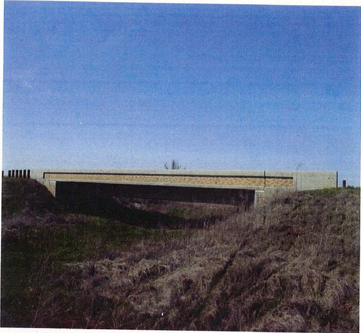
SOUTH YANKEE SLOUGH BRIDGE RIGHT - LOOKING WEST
